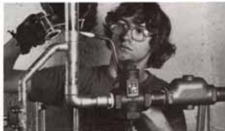
Air purger, valves and copper pipes were plumbed and soldered according to the manufacturer's recommendations.
