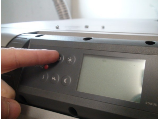
1. Shutdown the boiler.
