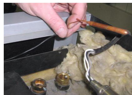
Bring the bulb to the back of the boiler
