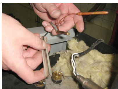
Prepare STL bulb and boiler temperature sensor
