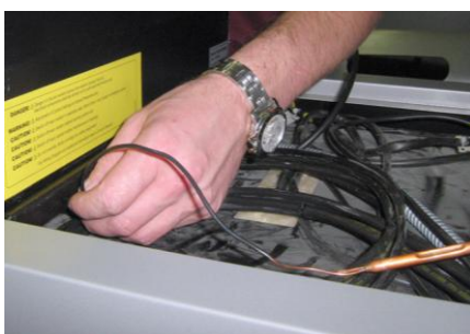
Feed bulb and capillary to back of boiler
