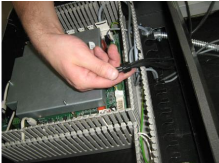
Feed Through Air Damper Wires
