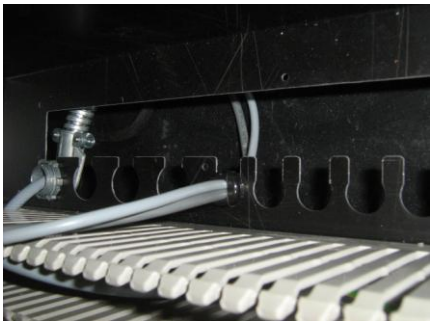
Feed Wires Through Wire Knockout
