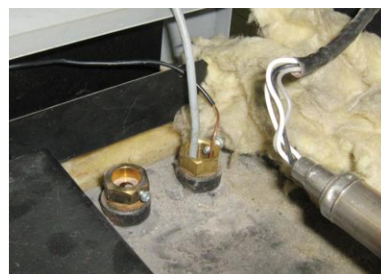
Make sure the sensors are pushed completely into well
