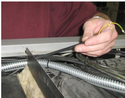
Feed through Flue Gas Sensor Wires
