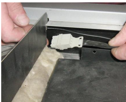
Feed through Lambda Probe Wires
