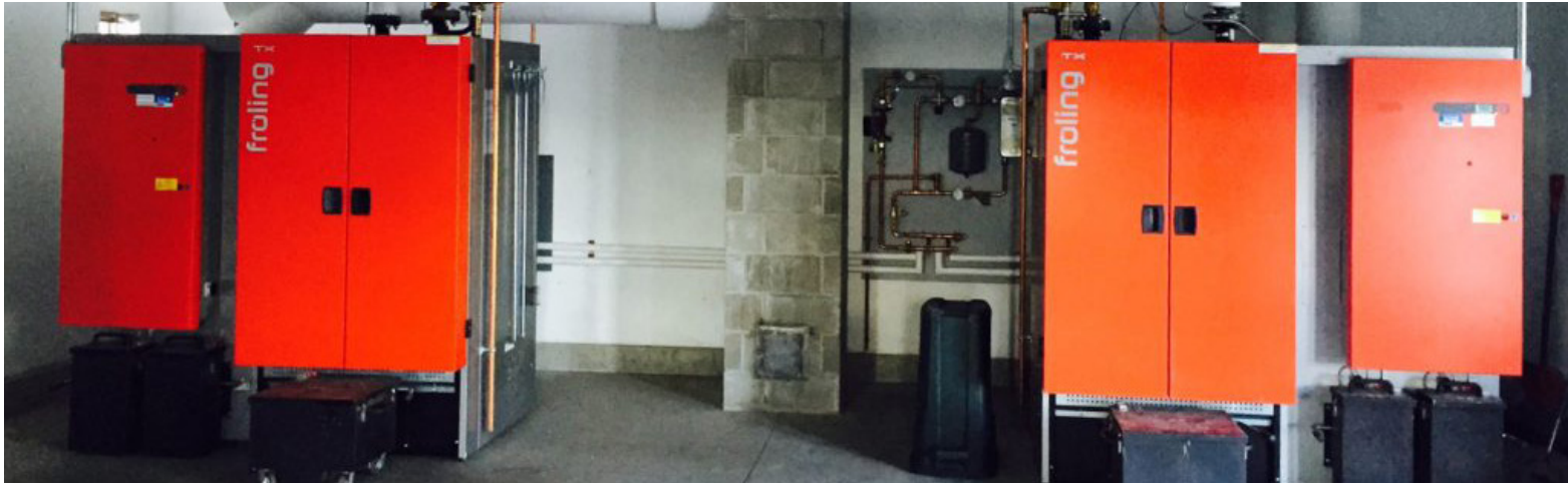
Two Fröling TX-150 Boilers
