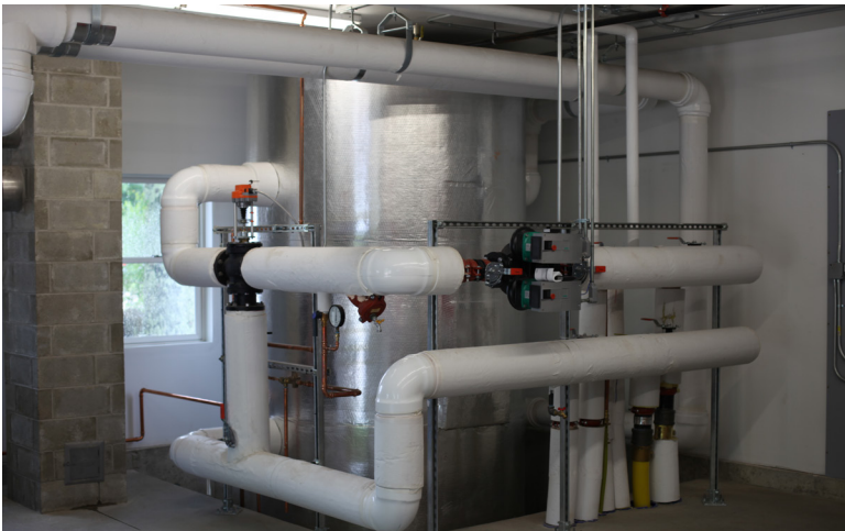
3000 Gallon Thermal Storage Tank
