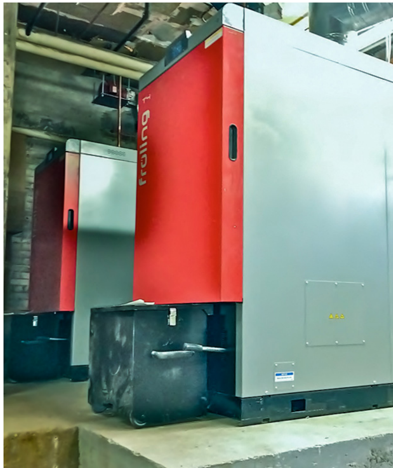
Two Fröling T4 150 wood pellet boilers
