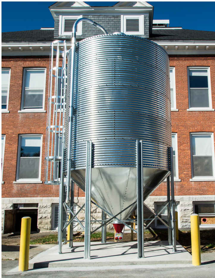
36 Ton Pellet Fuel Silo
