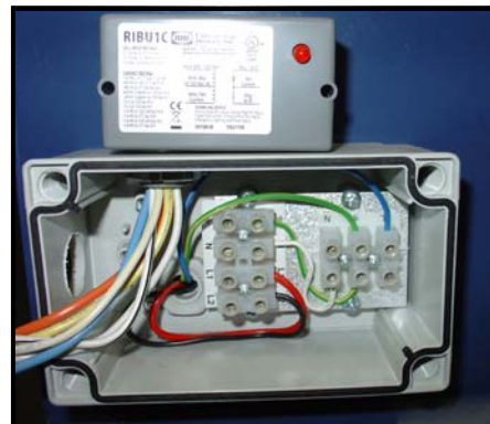
Fig. 3.15 Mounted RIB Relay
