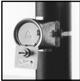
Barometric damper on vertical chimney
