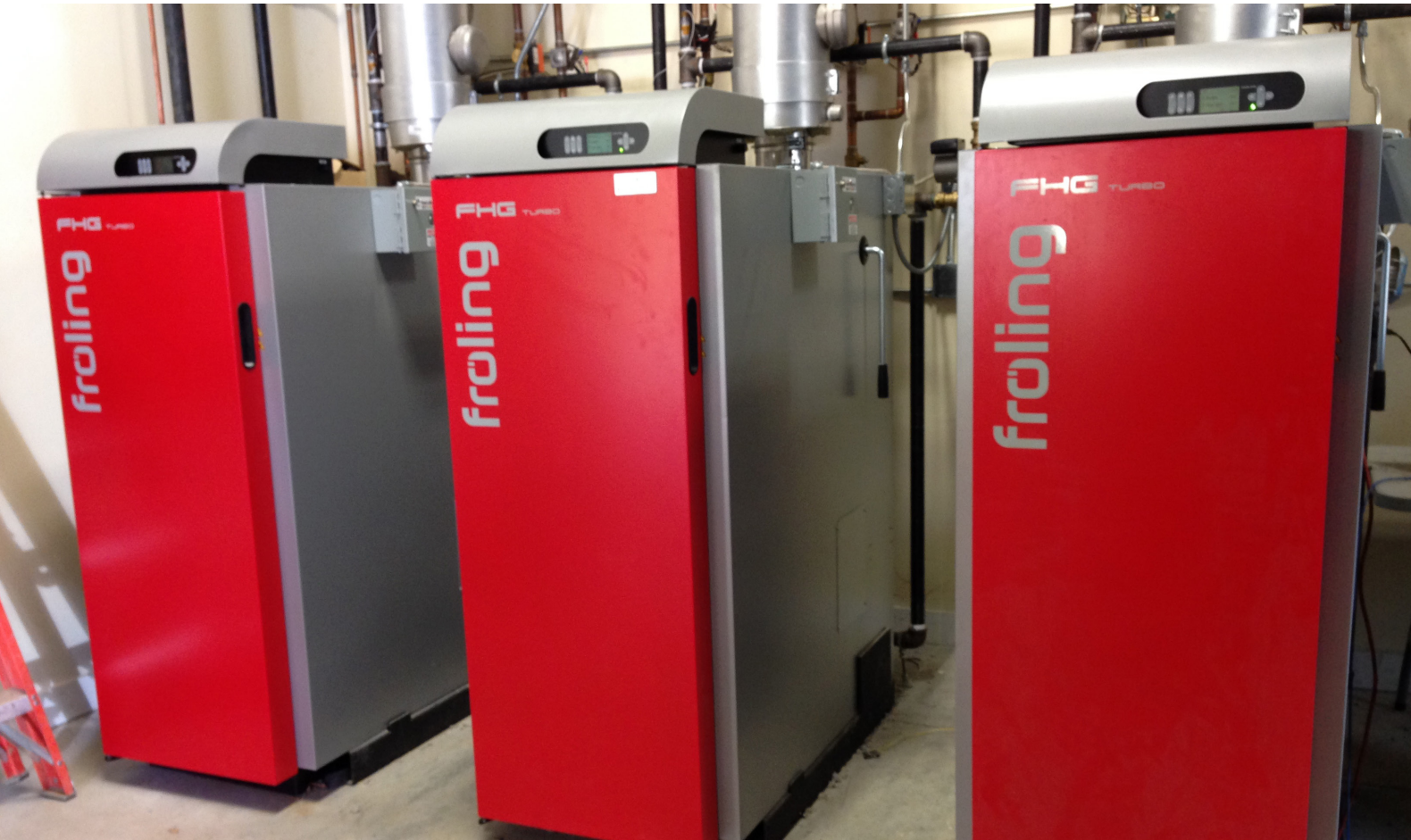
Three Fröling FHG 50 KW wood boilers
