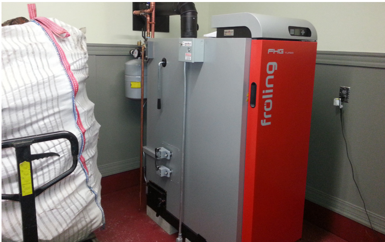
Fröling FHG 50 KW cord wood boiler.
