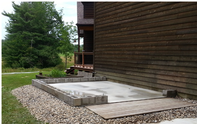
New pad for the boiler room.
