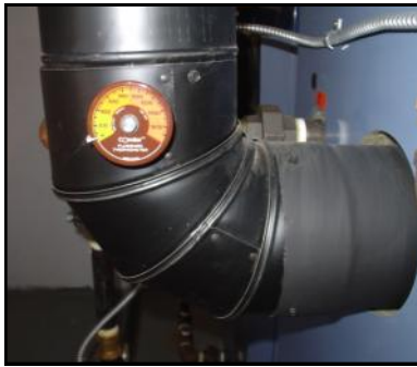
Fig. 3.5 339N Thermometer Installed
