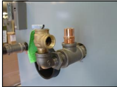
Fig. 3.6 Installed Relief Valve
