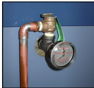
Fig. 3.10 Installed Relief Valve
