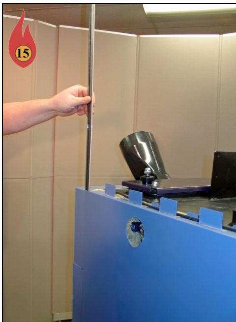
Install Left Rear Corner Zip Strip
