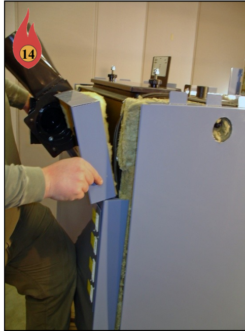
Place Upper Rear Panel into Place
