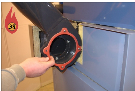
Place Fan Gasket on Housing
