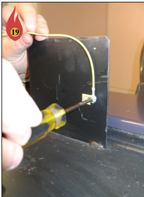
Install Ground Wire for Control Panel
