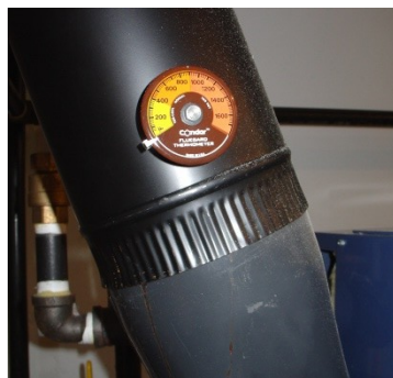
Fig. 3.5 339N Thermometer Installed
