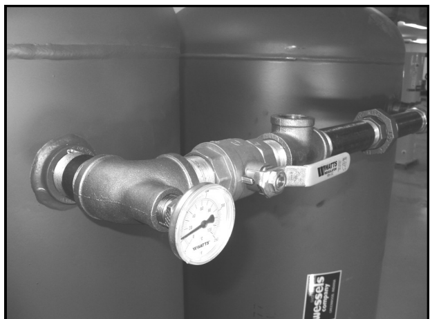
Completed Left Top Connections
