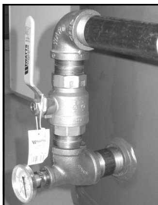
Completed Left Connections
