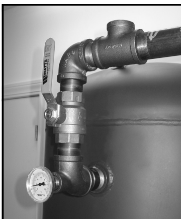
Completed Left Connections
