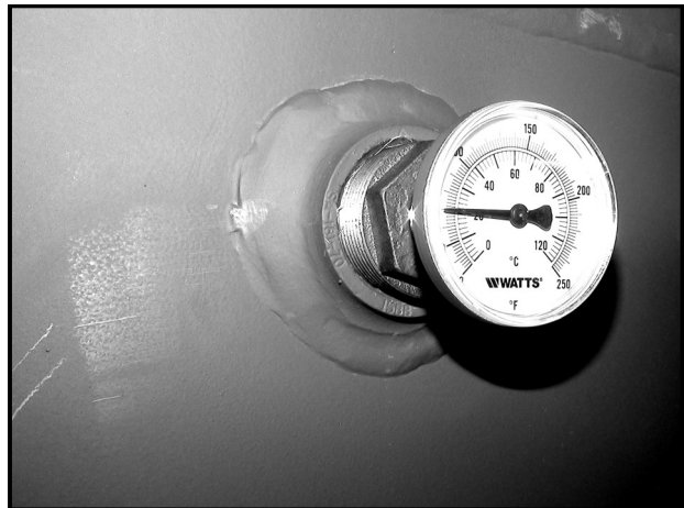
Install Temperature Gauge in Upper Tappings
