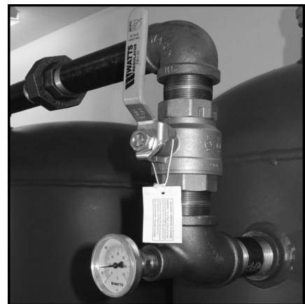
Completed Right Connections
