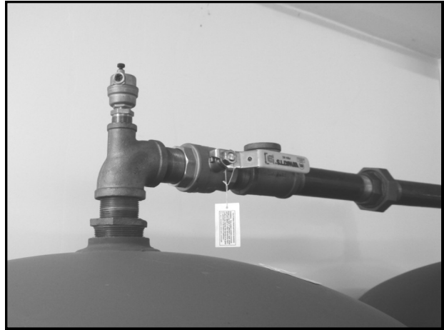
Completed Left Top Connections
