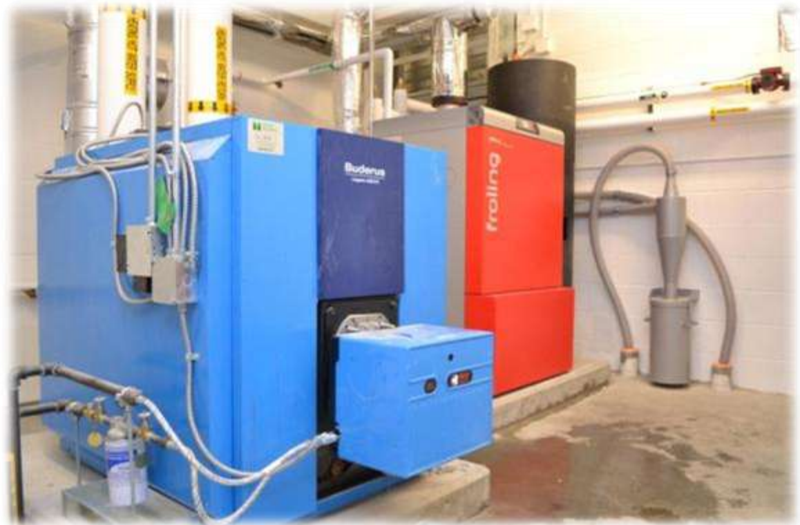
Peak and redundant load boiler
