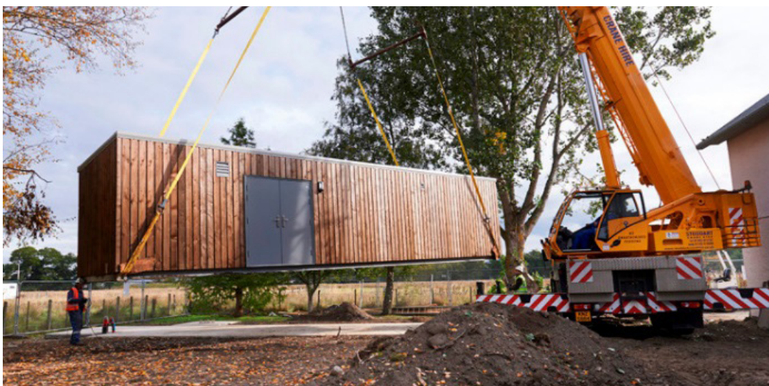
FIGURE 5 Installation of a containerized system
